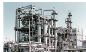
Chloroprene rubber plant (1971)
