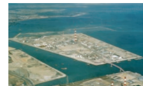
Kasumi Industrial Complex (1972)
