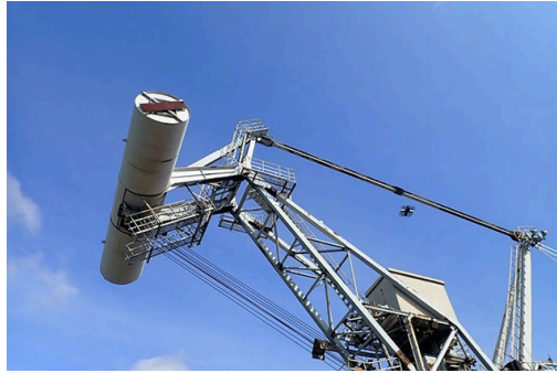
Drone-based visual inspection of elevated areas
