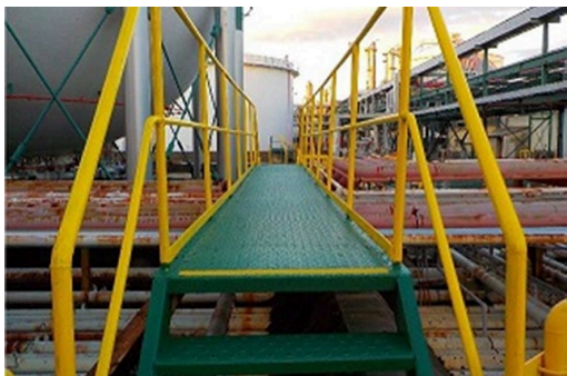
5S Activities: Painting safety corridors in-house (Yokkaichi Complex)
